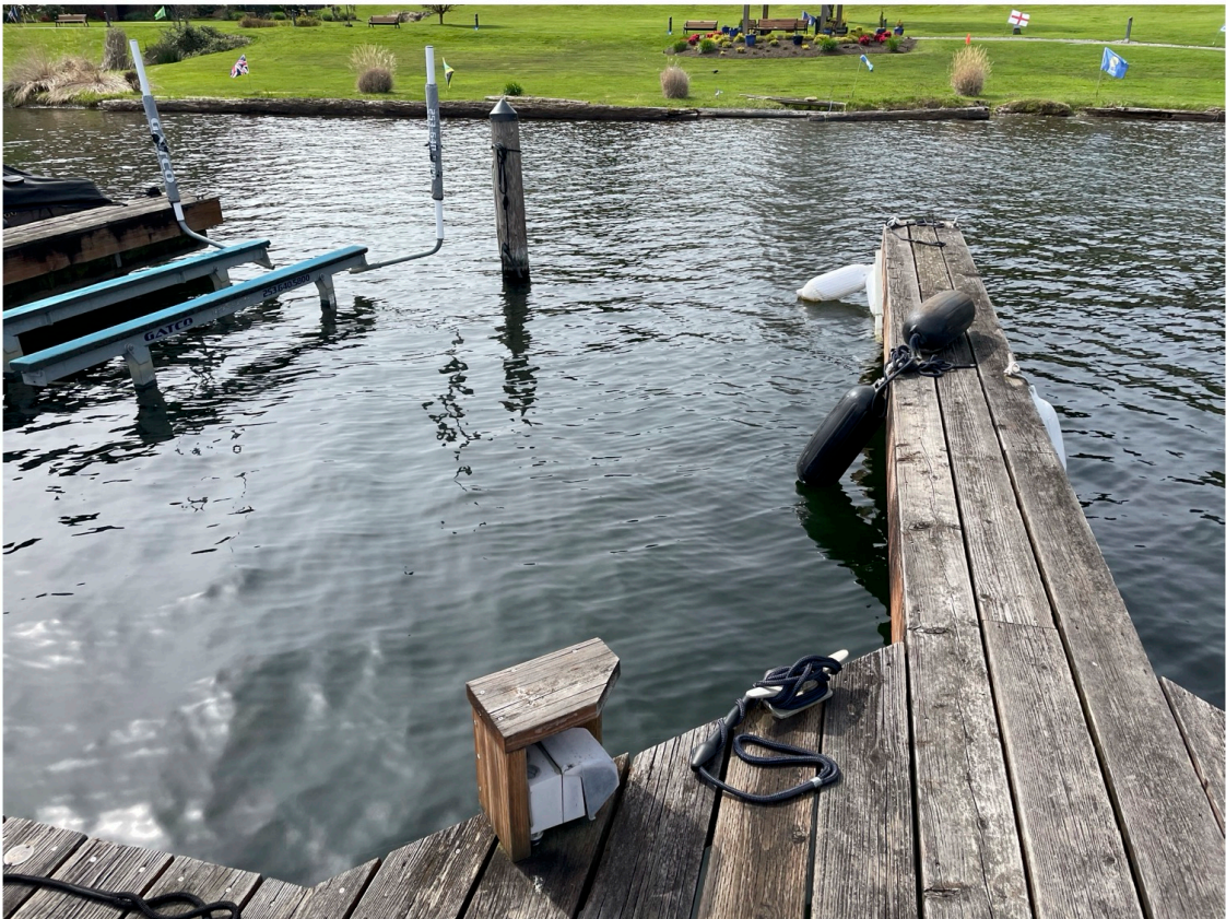
Photo 2 - Levitt slip existing conditions.
