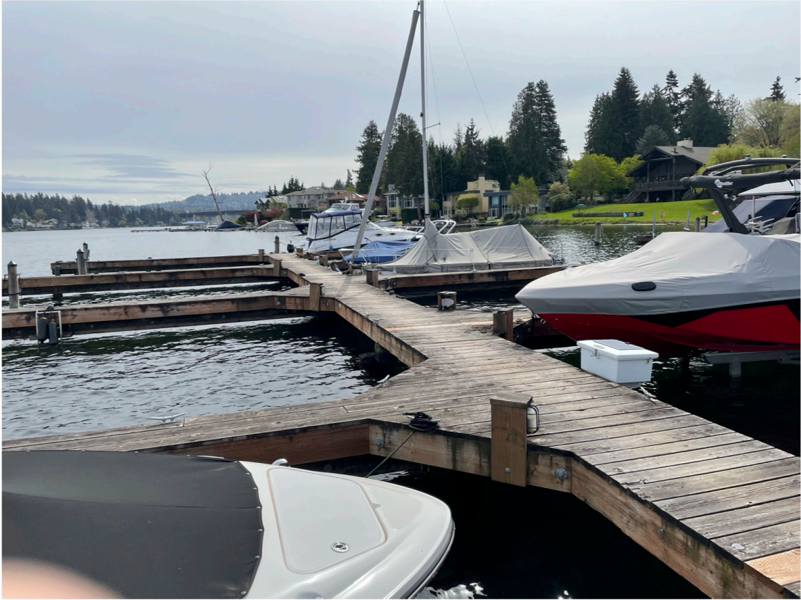
Photo 3 - Middle finger pier.
