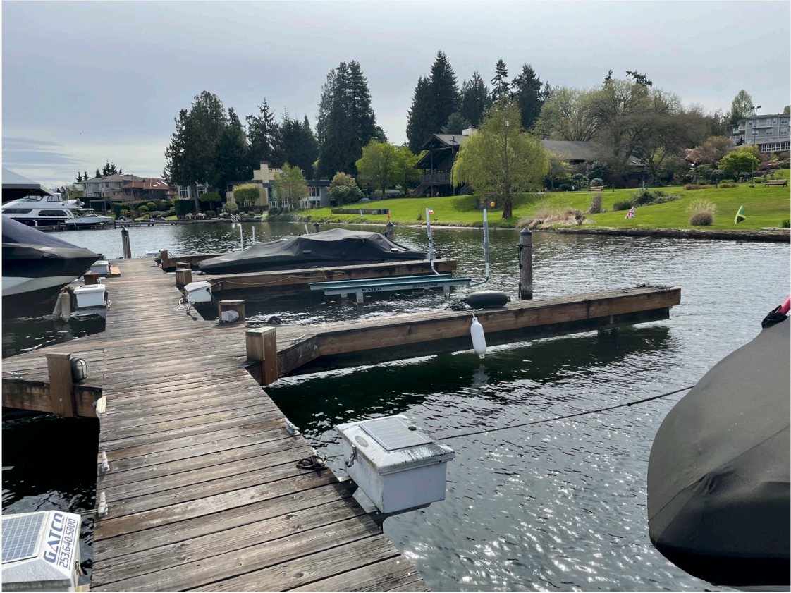
Photo 1 - Shoreward finger pier.
